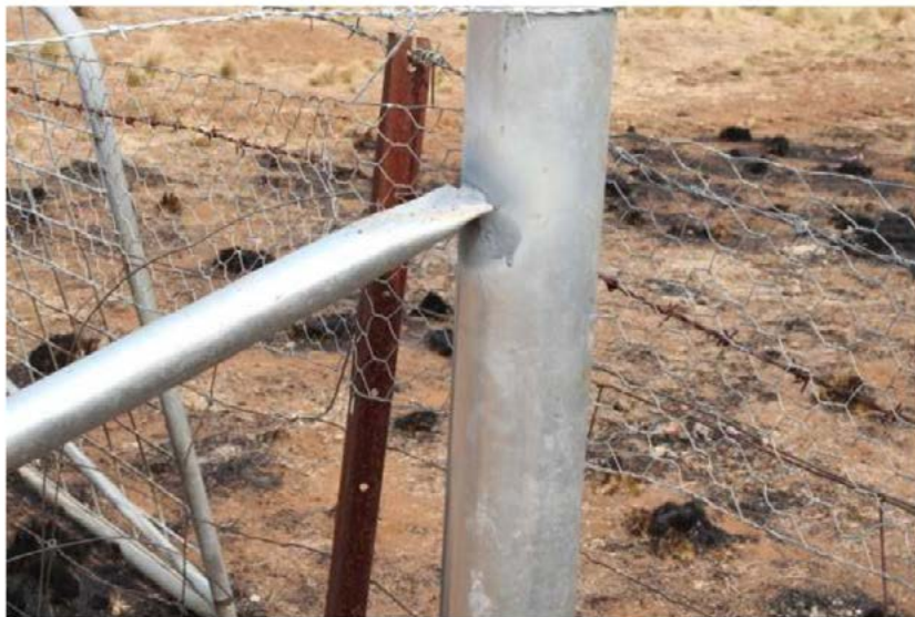
D021 Photo from Kevin Pearce - Strainer post that has been welded at the origin area
