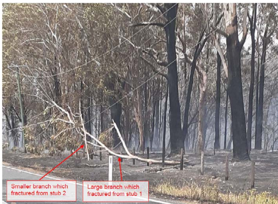
Figure 7 Fallen branches suspended on powerline below the Subject Tree
